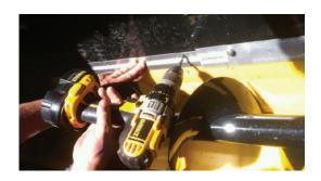
6. Install stainless hold down strips, using either the pop rivets or the self drilling screws. Start on one end and work your way to the other end. Proceed to the next hold down strip after you finish the first. If using pop rivets drill 13/64 hole as shown left then insert rivet as shown below before moving on to the next hole.
